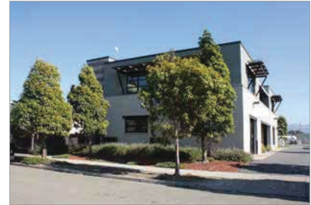
Existing industrial buildings in the Seaport area
