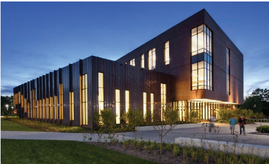
Large expanses of glass should be focused on entries and other key public building functions and shaded appropriately.
