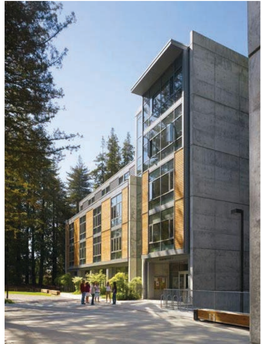
The combination of materials - precast concrete, glass, and tastefully-colored aluminum - is successful on this lab building (left). Wood infill can be used to soften the appearance of poured-in-place concrete (right).
