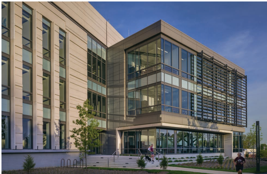
The combination of materials - precast concrete, glass, and tastefully-colored aluminum - is successful on this lab building (left). Wood infill can be used to soften the appearance of poured-in-place concrete (right).
