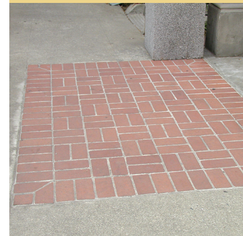
Example of a basket-weave pattern at a building entrance (2003).
