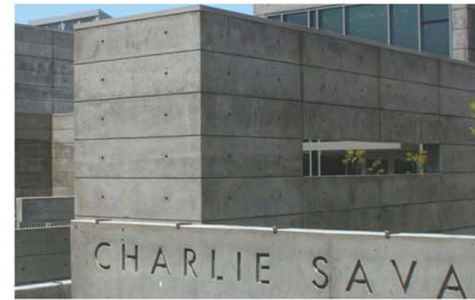
CONCRETE WALLS - BOARD FORM FINISH
