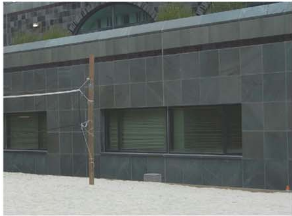
EXISTING FACADE - SODA HALL
