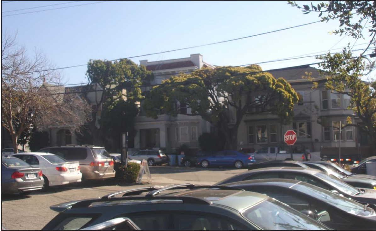
Photo 5 - View of residential buildings across Durant Avenue from the interior of the project site.
